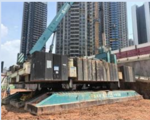
“静压桩机+边桩器”边桩施工
