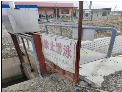
渠道现状分水闸
