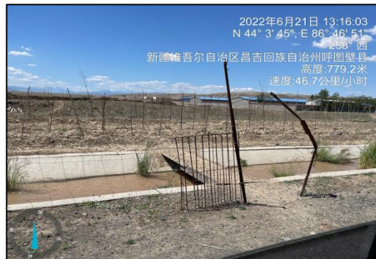
渠道现状桥涵
