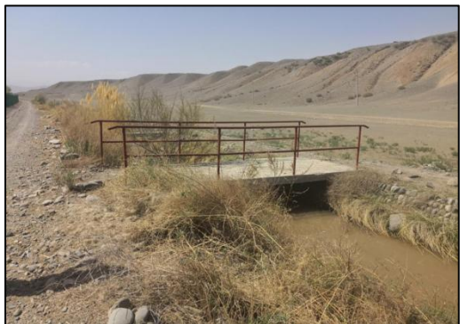
渠道现状桥涵
