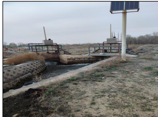
渠道现状分水闸和桥涵
